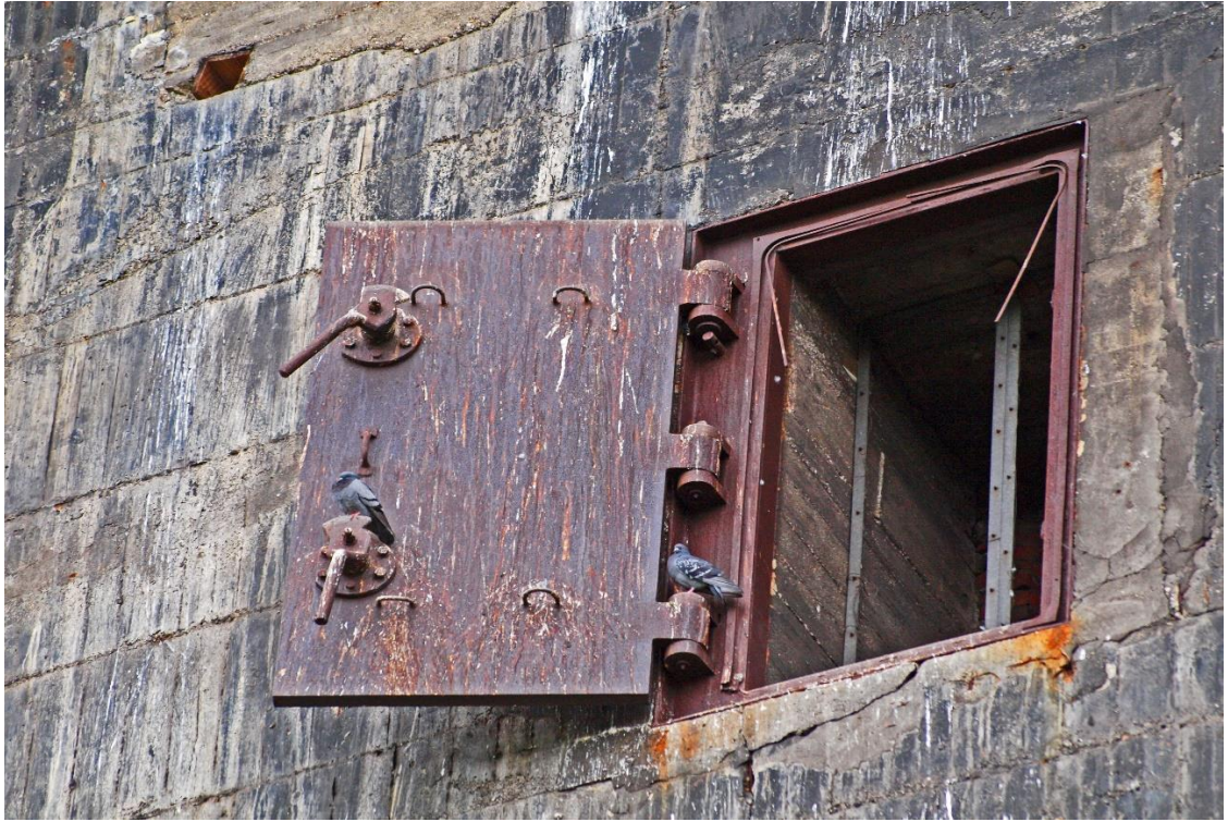
Bunkertür © Uwe Duwald / pixelio.de
